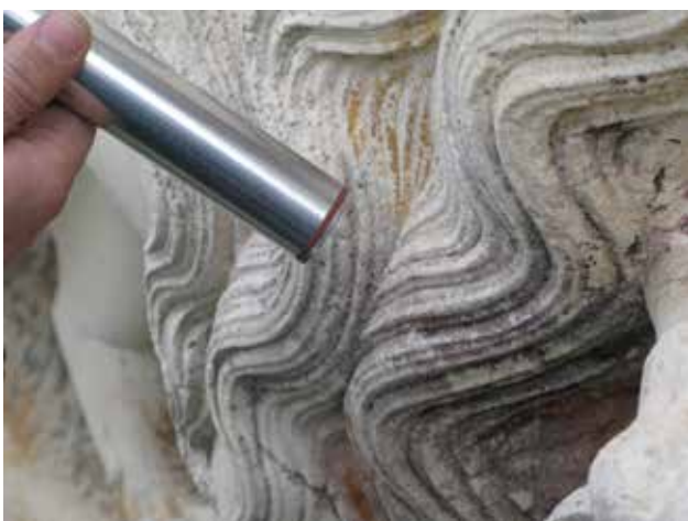
25 Detalj čišćenja kamene plastike laserom (foto: P. Ajduković, 2013.) Detail of laser cleaning of stone plastic (photo: P. Ajduković, 2013)
