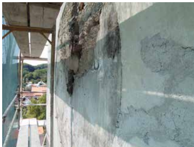
19 Pozicija na zvoniku crkve sv. Martina biskupa u Varaždinskim Toplicama s koje su skinute ploče sata, nazire se stariji, pismoslikarski izveden sat, stanje tijekom obnove 2011. godine (foto: M. Korunek) Position on the belfry of the church of St. Martin the Bishop in Varaždinske Toplice from which the plates of the clock have been removed, an older cock painted on the wall may be discerned, condition during restoration, 2011 (photo: M. Korunek)
