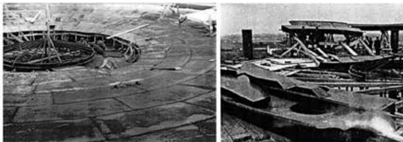
11 Izvedbeni nacrt prstena, 1936.; varenje prstena i limenih ploča, 1937. (Muzej arhitekture, Arhiva materijala o Francuskom paviljonu) Implementation design of the ring, 1936; welding of ring and metal sheets, 1937 (Museum of Architecture, Archives of materials on the French Pavilion)
