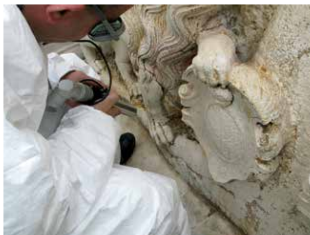
26 Čišćenje laserom središnjeg reljefa s dvama lavovima i grbovima, stanje pri dovršetku zahvata (foto: P. Ajduković, 2013.) Laser cleaning of central relief with two lions and coats of arms, condition at the end of the intervention (photo: P. Ajduković, 2013)
